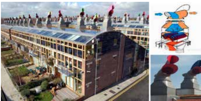
Figure 3. Rooftop ventilation system [17]
