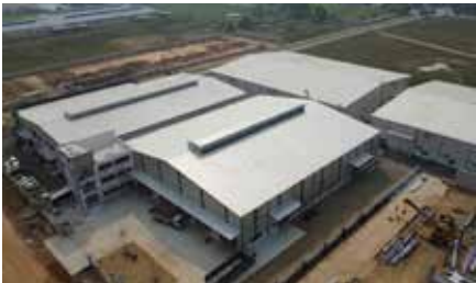
Figure 1. Large-span industrial factory building
